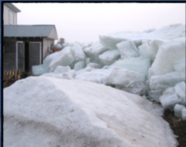
May 30, 2011 - Sea Ice Kotzebue, AK structure damage
